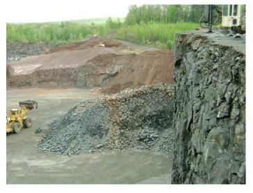
shot readings were .09ppv @ 18hz, which is typical for this area.
